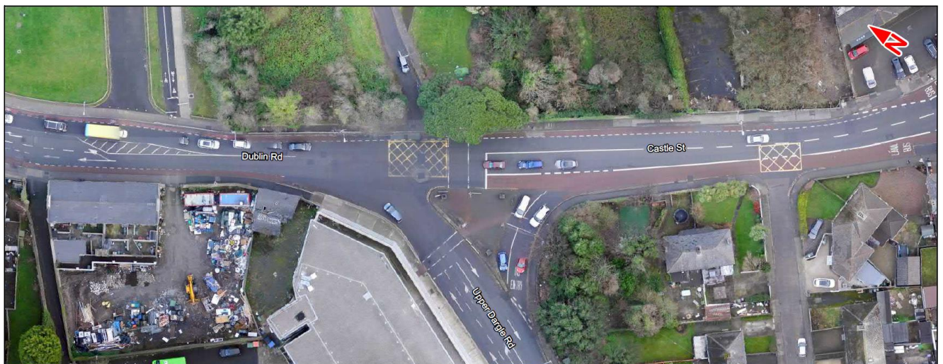
Image 5.46: R761 Dublin Road / R918 Upper Dargle Road Three-Arm Signalised Junction
