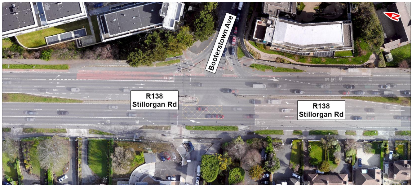
Image 5.22: R138 Stillorgan Road / Booterstown Avenue Three-arm Signalised Junction
