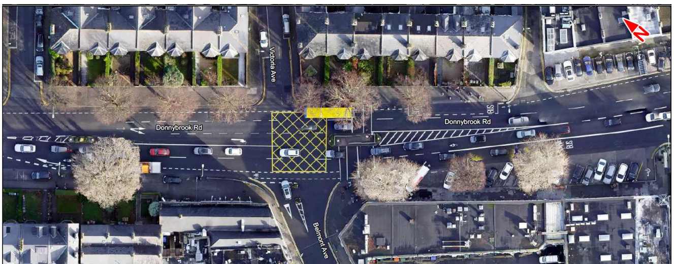
Image 5.12: R138 Donnybrook Road / Belmont Avenue Priority Junction
